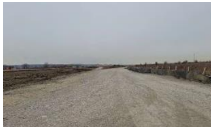
Placement and compaction of granular
