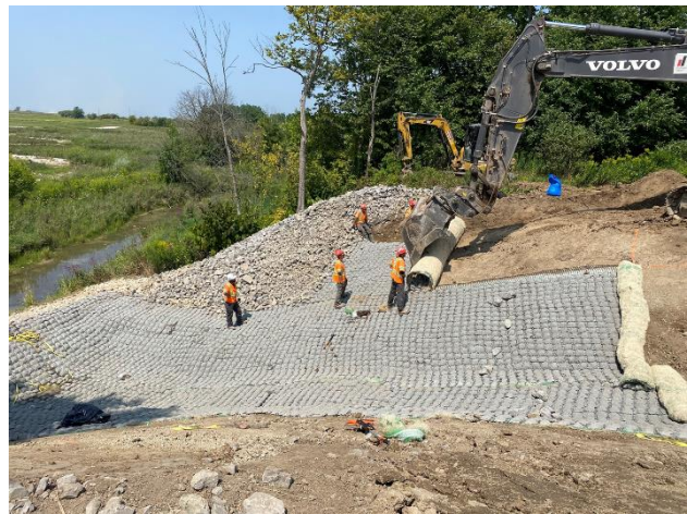
Image 2: Installation of Terrafix Flexamat protective barrier
