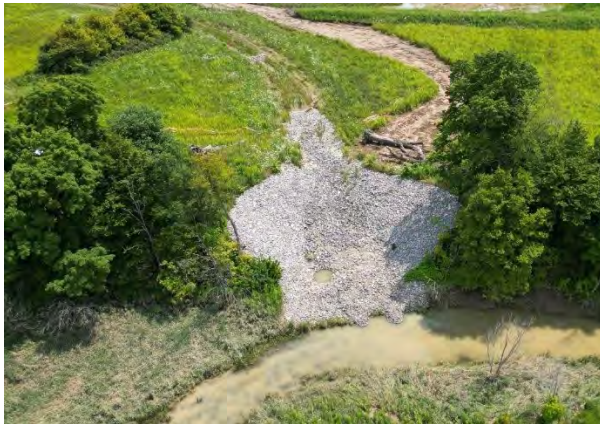
Photo 5: Temporary repair to the spillway
