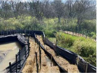
Photo 4: Installed of double row of strawbales
