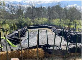
Photo 6: Installed filter fabric liner and filter bag in sediment basin
