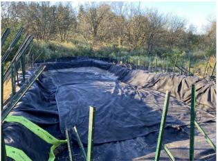
Photo 7: Installed 10 m filter bag in sediment basin
