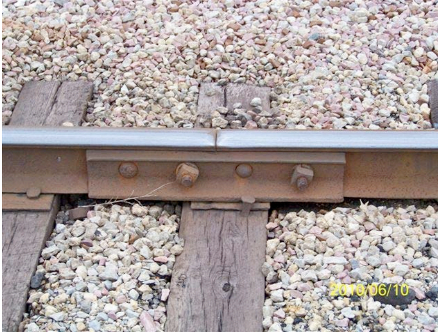
(Figure 14: Tie at joint)
