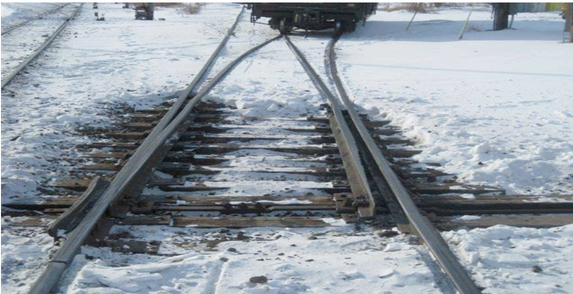
(Figure 24: Cleared switch)
