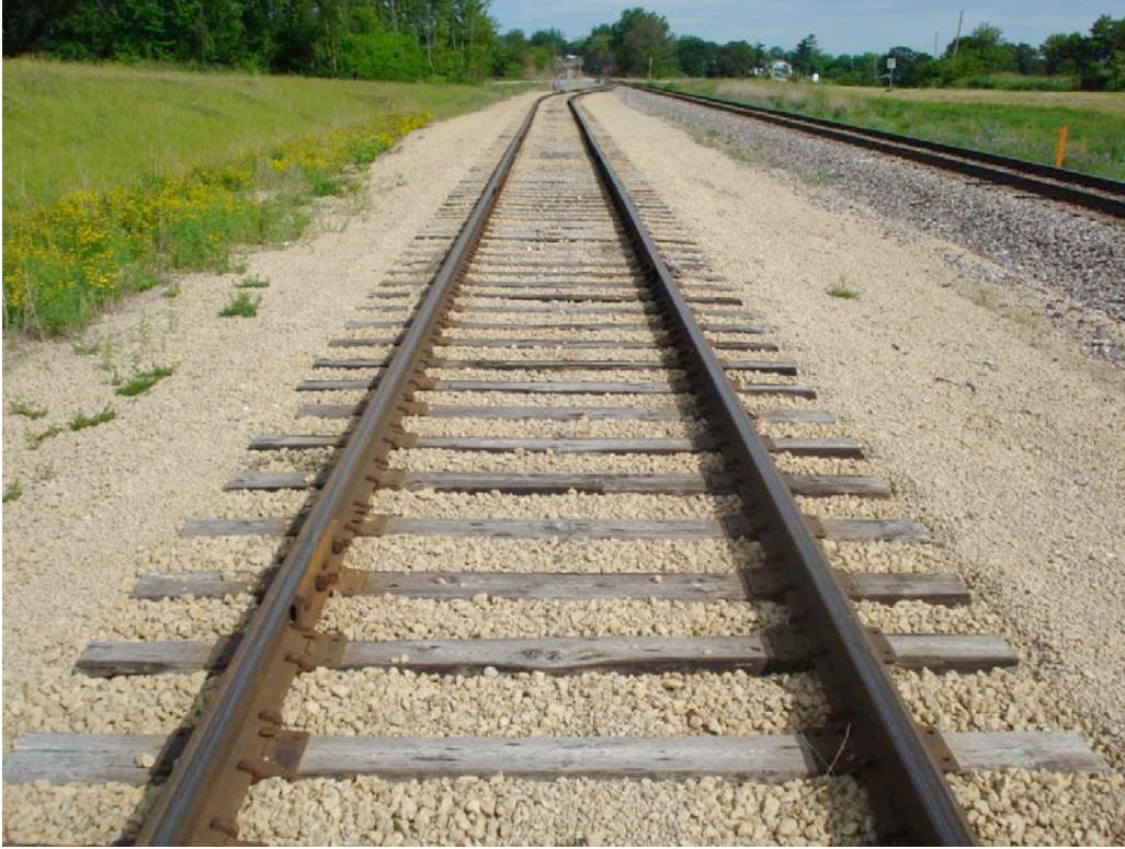
(Figure 11: Clean ballast)
