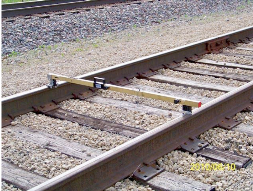
(Figure 8: Track level)
