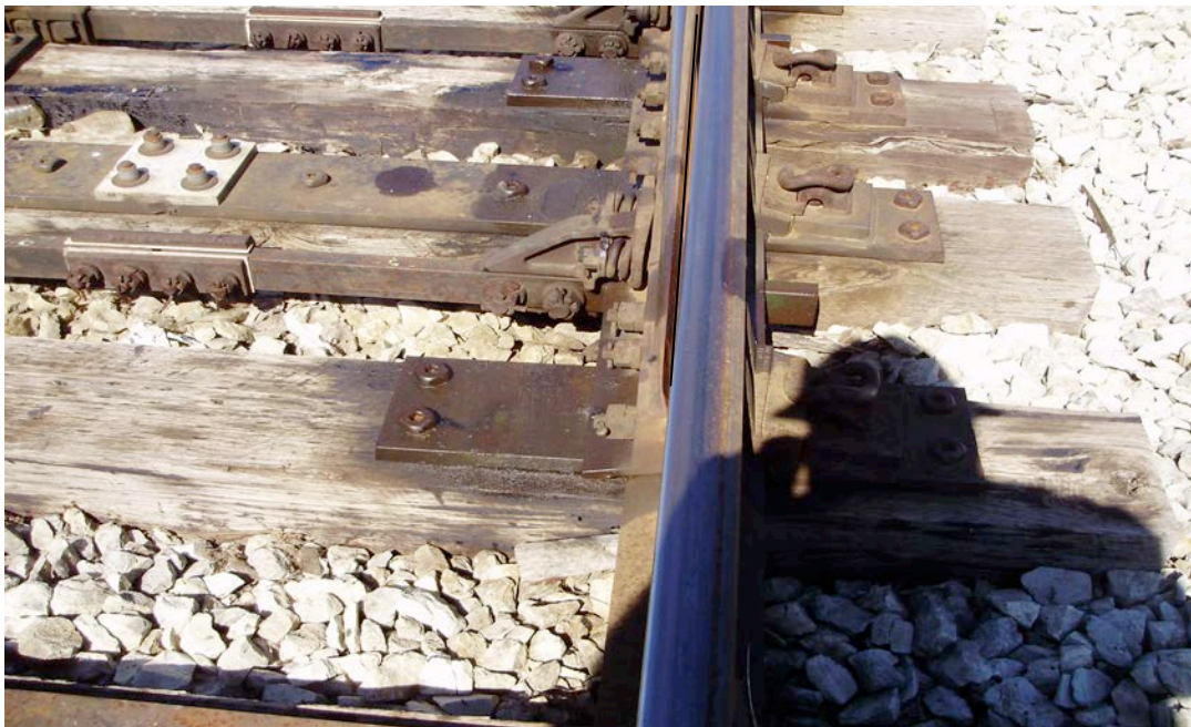
(Figure 22: Gapped Switch Point)
