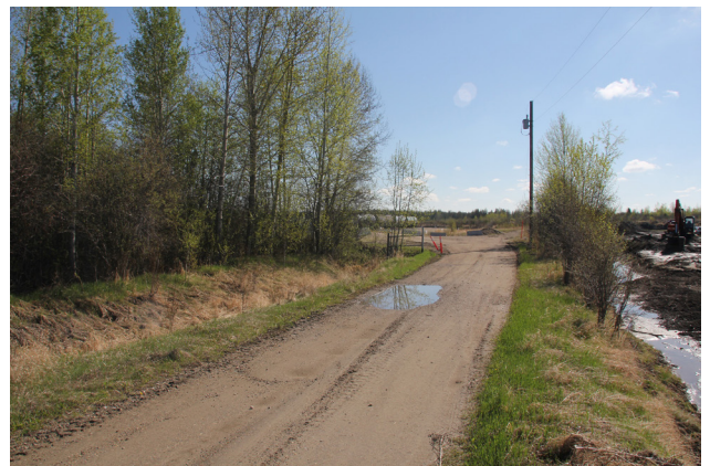
Southwest corner access road
