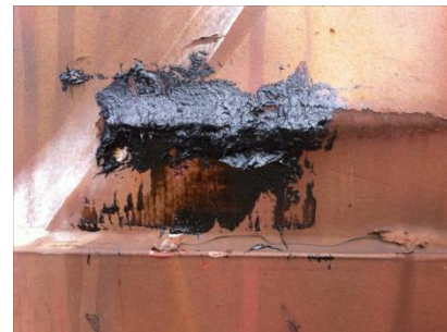
Roofing cement repair
