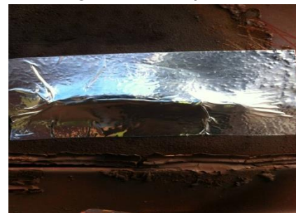
Silver/rubber seam tape repair
