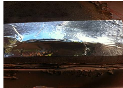
Silver/rubber seam tape repair
