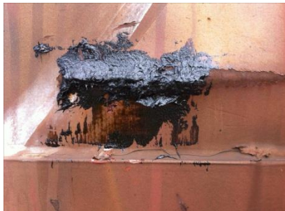
Roofing cement repair
